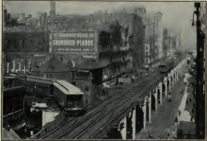
FIG. 262 — A view of an elevated railway in Chicago at the point known as the Union Loop.
